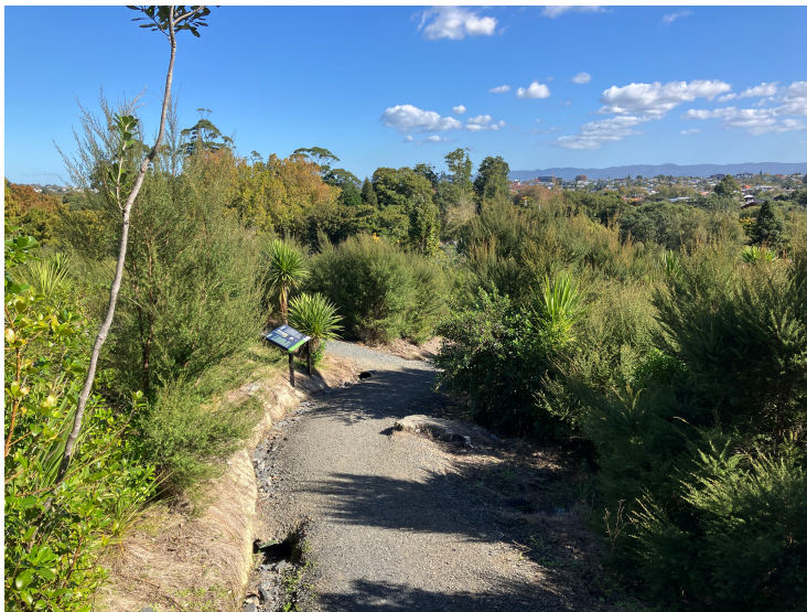
The flourishing revegetation planting, new walking track, and interpretation signage at Western Springs.
